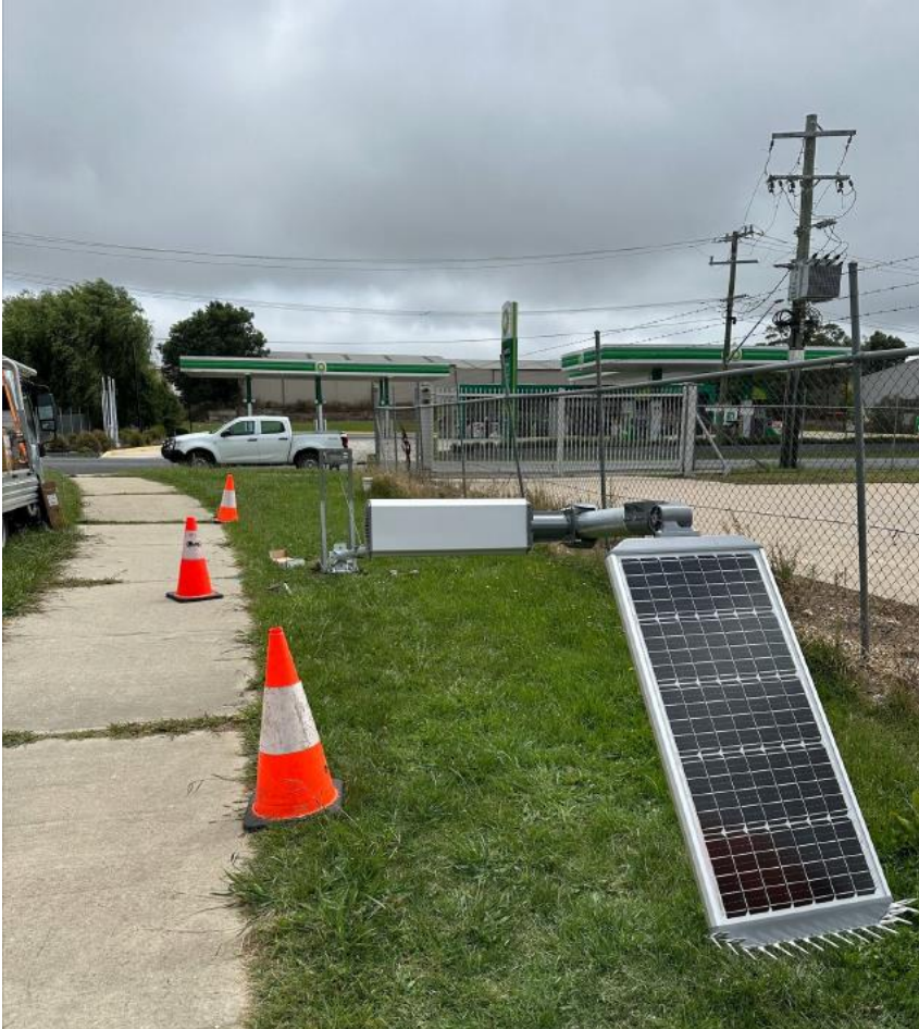
Solar lights going up between Oberon High School and Albion St
