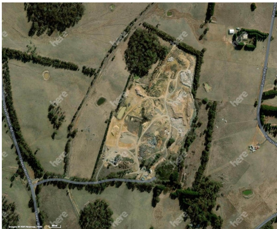
Figure 3 – The Oberon Waste Facility
