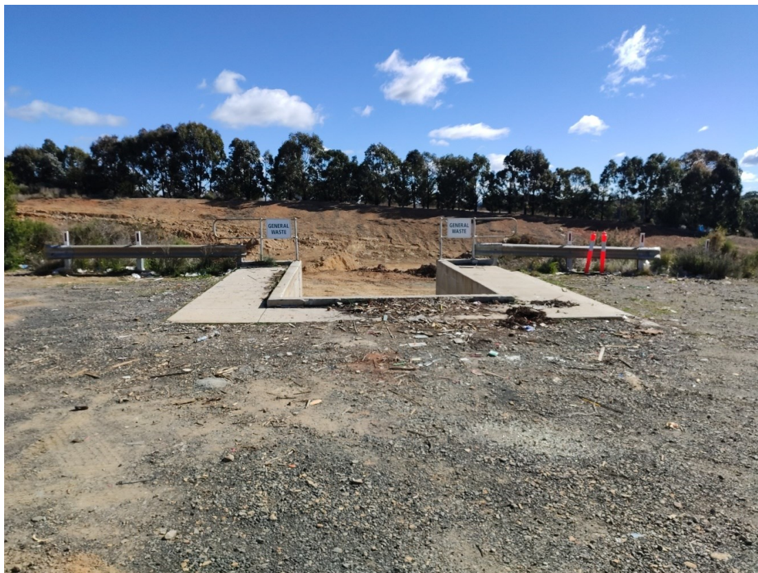
Photograph 19 – Small vehicle facility (Location 22)
