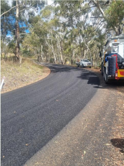
Pothole patching on Sewells Creek Road.
