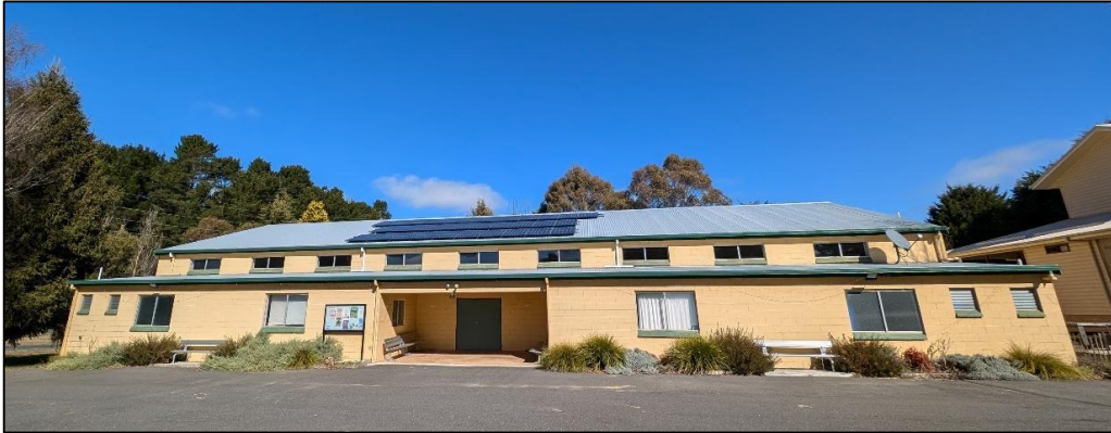
Figure 19: Black Springs Hall (existing 10kW solar PV)
