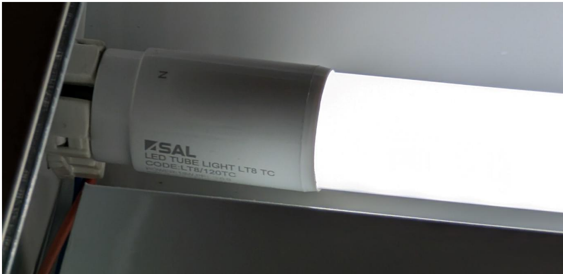
Figure 12: Council Admin - LED Tube Replacement
