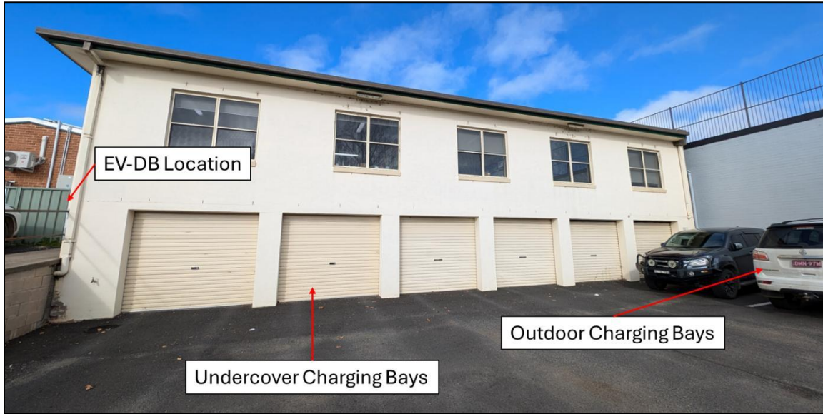
Figure 9: Indicative EV Charging Layout
