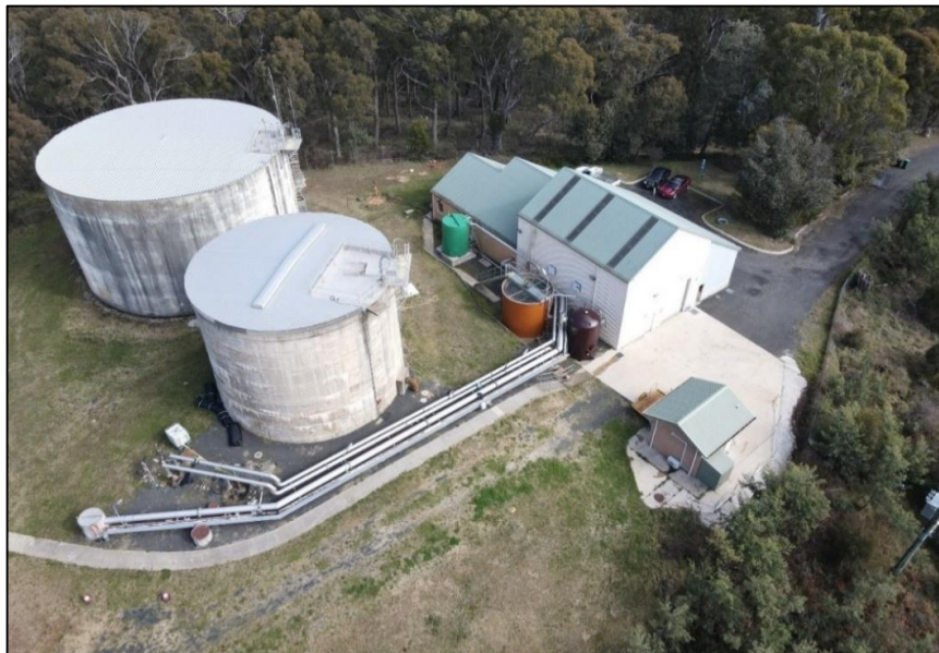
Figure 2: Water Treatment Plant
