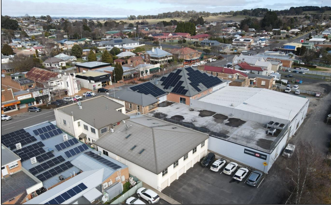
Figure 6: Oberon Council Administration Building
