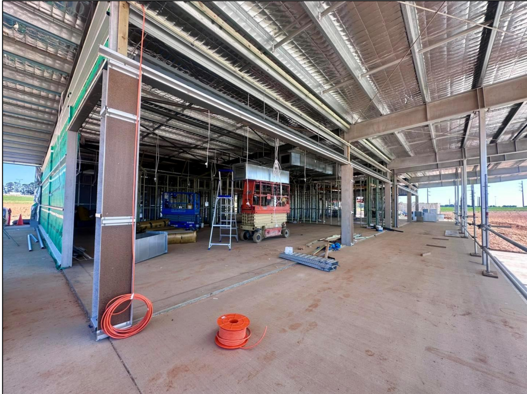
Figure 22: Sporting Complex Site
