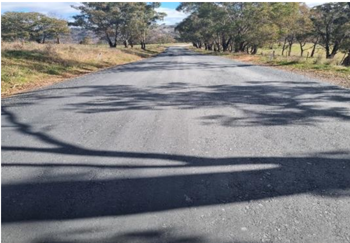
Figure 2: Sewells Creek Gravel re-sheeting works, approximately 1.3 km
