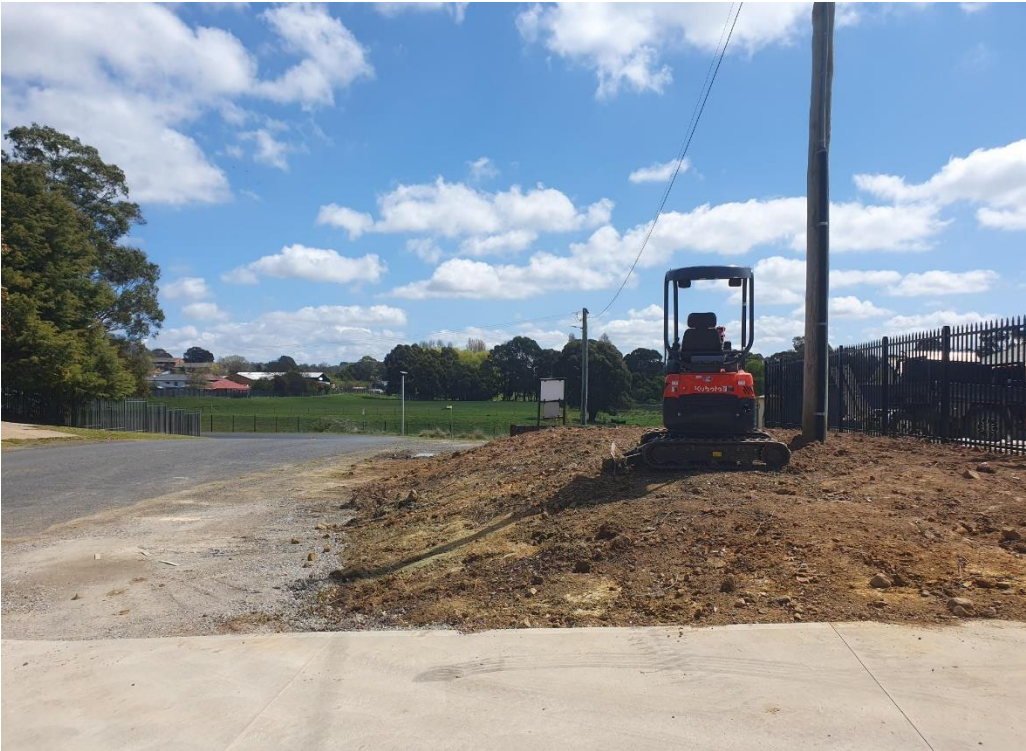
Figure 4 showing street alignment to the west (3 Oct 2024)
