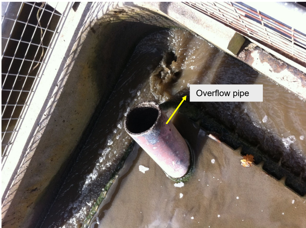
Figure 4.2 Photo STP Aerator Tank
